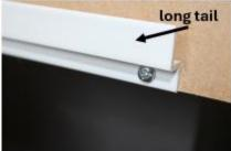
Note: If the track does not butt up to a wall/frame you can use the stopper provided. Insert the stopper between the tail of the track and your frame and secure with the end screw in each case.
